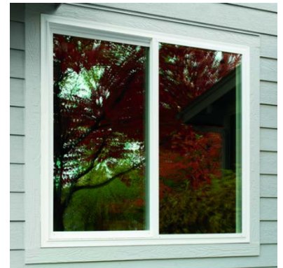
Windows: Vinyl extruded dual pane insulated low E windows
