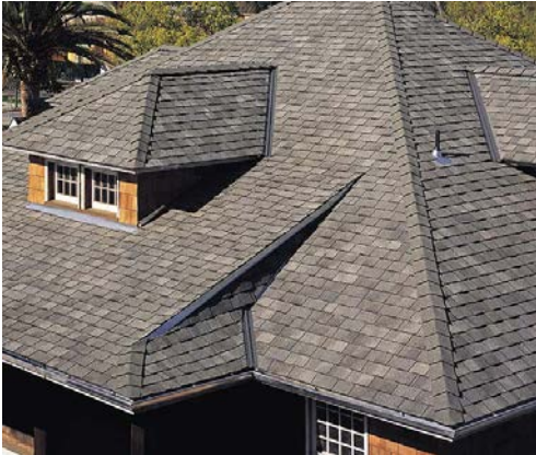
Roof: 30 year architectural asphalt Composite shingles
